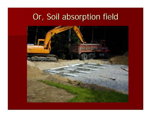
Once in the drainfield, the wastewater flows out of the perforated pipes into the stone bed below, where it pools for a wile and allows more bacteria and microbes to continue to digest the suspended solida that have washed out of the tank.
